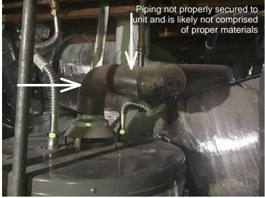
4. Crawl space Water Heater TPRV and Drain Tube: Copper - The TPRV currently takes a 90 degree bend shortly after leaving the unit. Its drain tube also has a very narrow slope exiting toward the exterior of the home. Recommend that this piping face directly downward and terminate within 6 inches of the crawl space floor.
